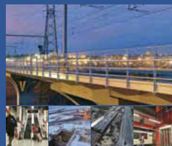
Images of the Northern Diabolo Project, completed during the six months to 30 June 2012.
