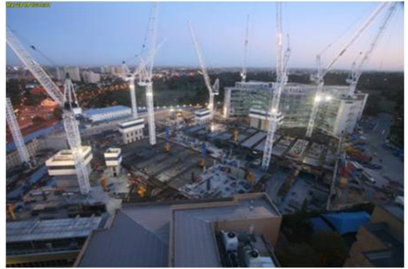
Construction status view (Mid 2010)
