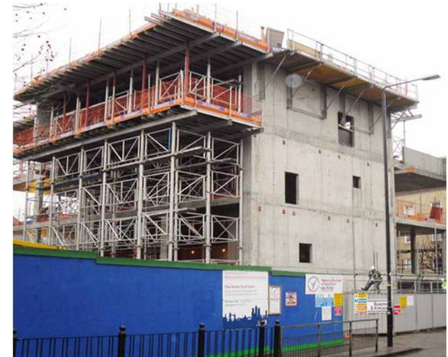
Construction underway at Osmani Youth Centre, Tower Hamlets (January 2011)
