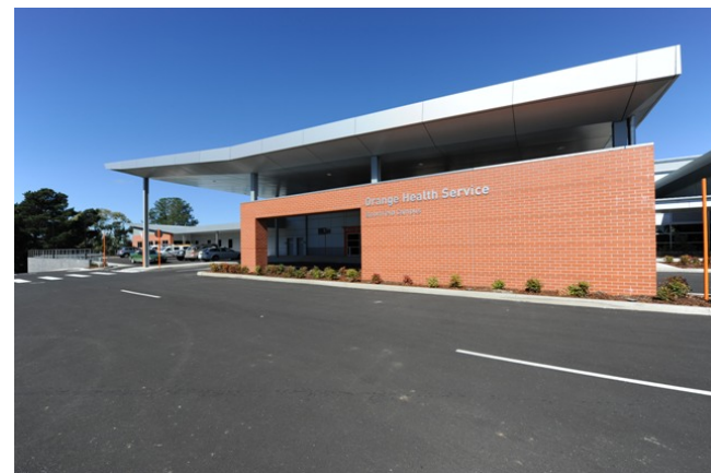
Orange Hospital, Australia
